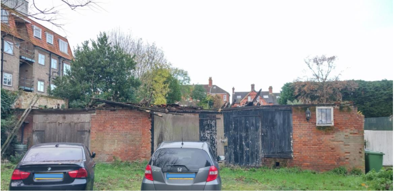
Fig2. Photograph of existing outbuilding
