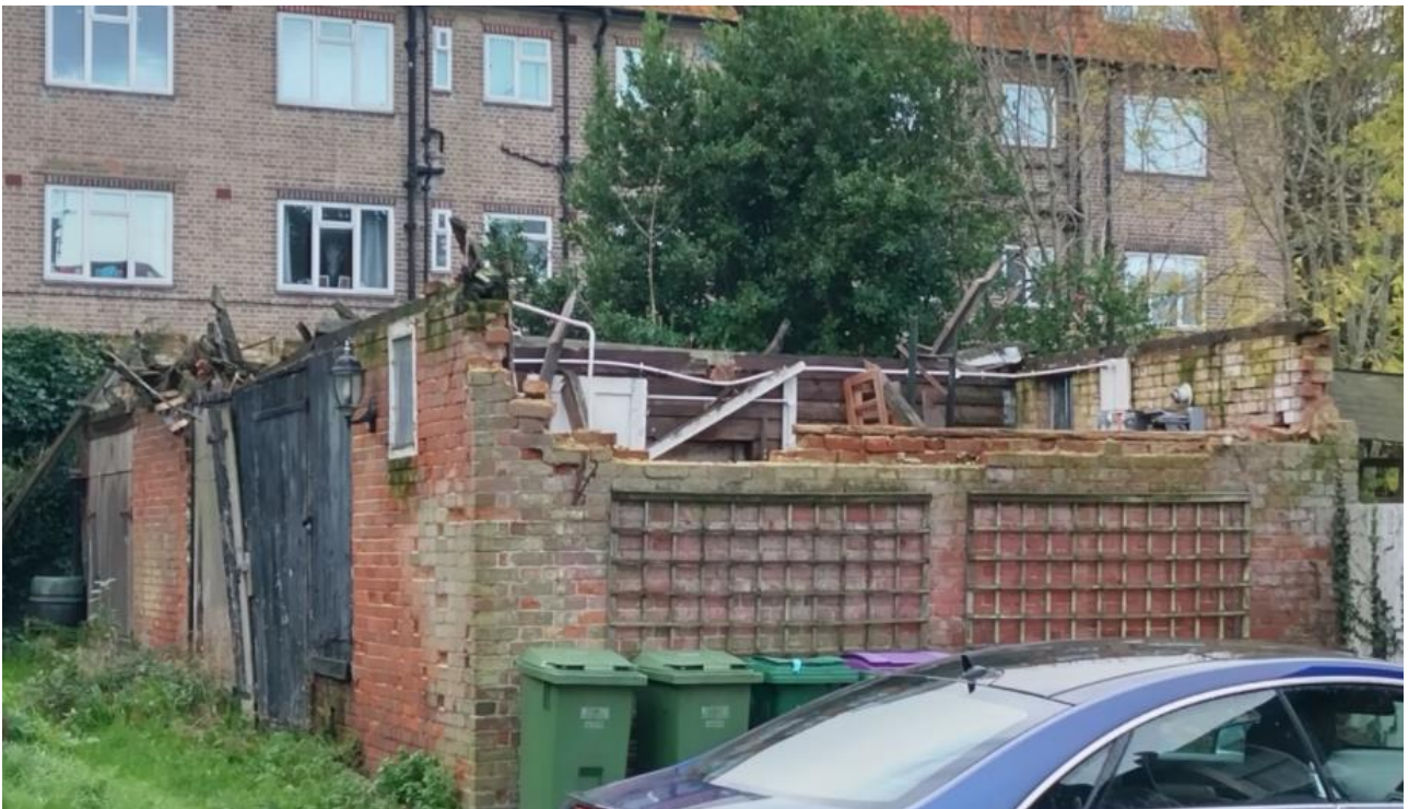
Fig3. Photograph of existing outbuilding
